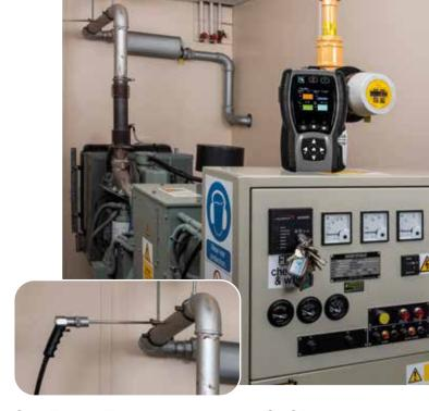
Gas Engine Testing with optional CHSP5 probe
